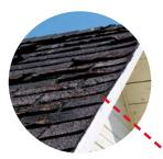
Missing, cracked, or curling shingles Possible cause: Shingles have reached the end of their useful life
