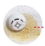
Stains on interior ceilings and walls or mold and mildew growth Possible causes: Inadequate or faulty shingle underlayment allowing leakage; inadequate ventilation
