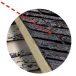
Roof shingle, sheathing, and siding decay Possible cause: Poor attic ventilation
