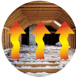
Excessive energy costs Possible cause: Insufficient attic ventilation causes heating/cooling system to run excessively
